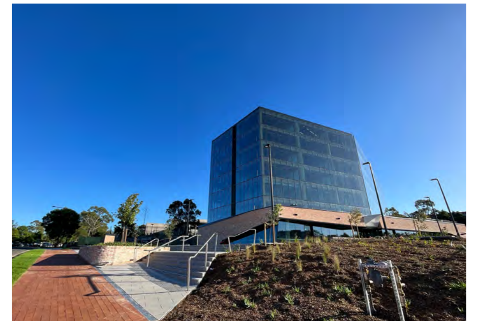
The completed project, view from Elizabeth Macarthur Drive
